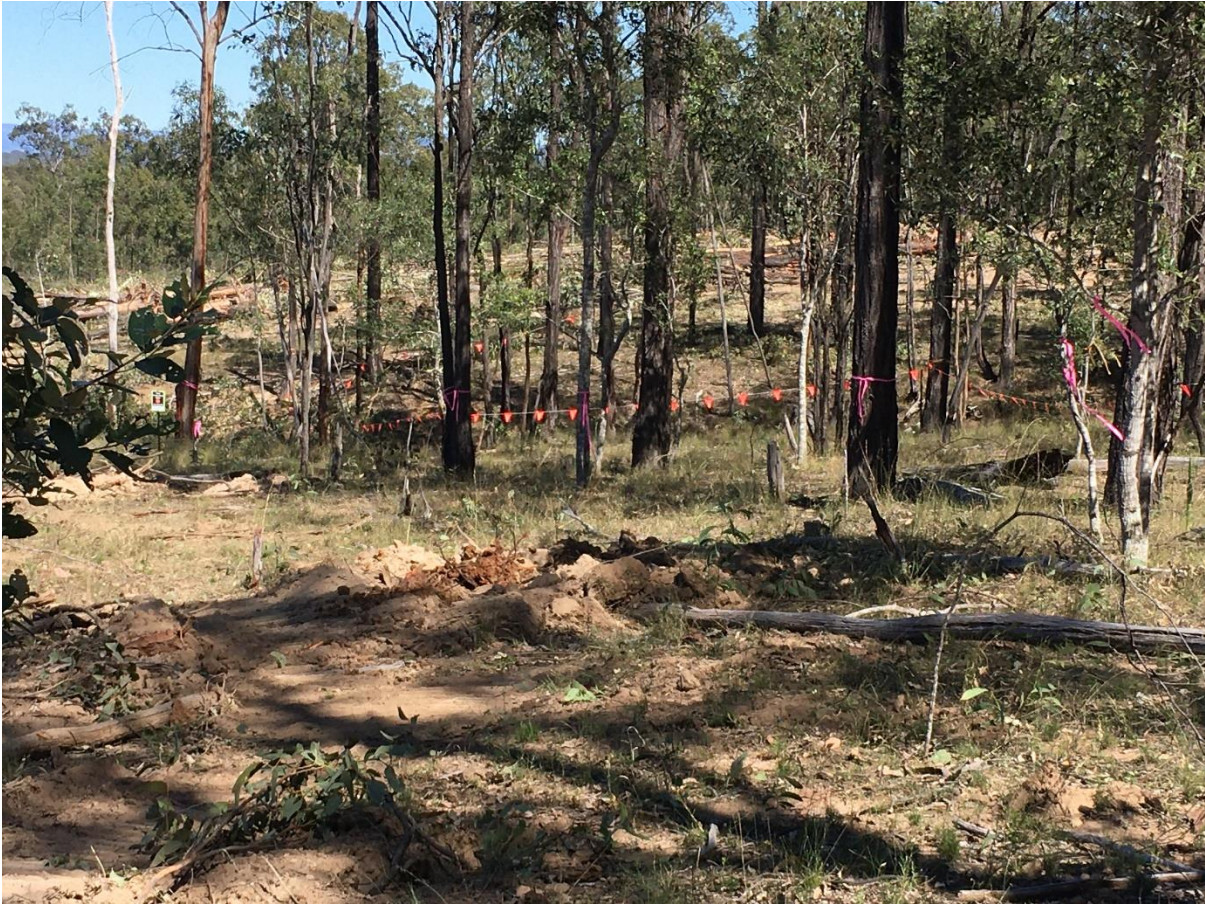
A buffer zone was created to allow works to proceed without impinging upon the TPZ.
