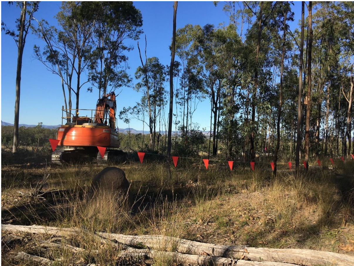
TPZ line demarcation was installed prior to any vegetation removal program.
