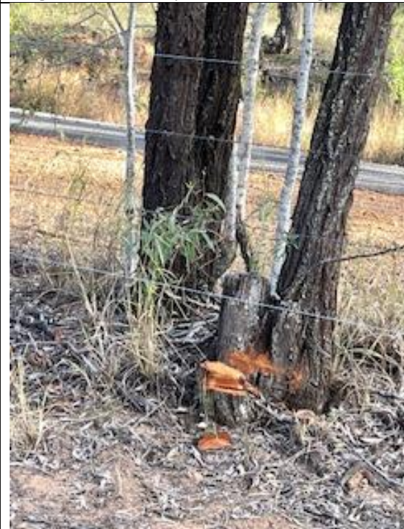
Removal of saplings to permit re-tensioning of fence along Rangers Road
