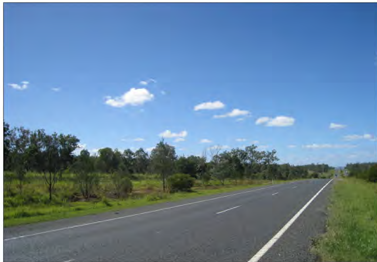
Site Photo - May 2009
