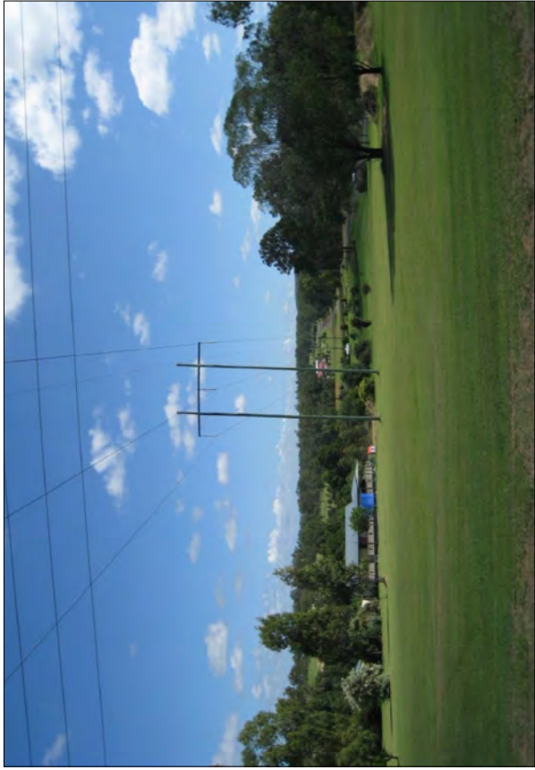
Site Photo - May 2009
